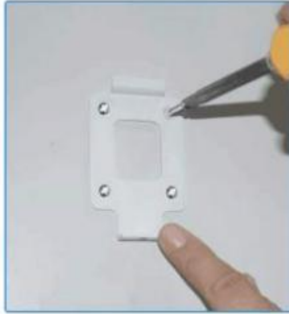
Drilling at a determined location Then fix the base with screws
